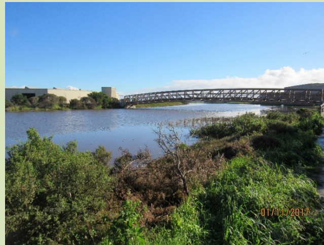
San Francisco Bay Trail pedestrian bridge – downstream end of project reach
