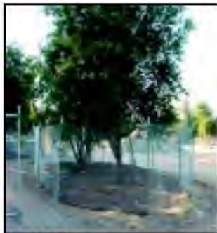
IMAGE 2.15-1 Tree Protection Fence at the Dripline
