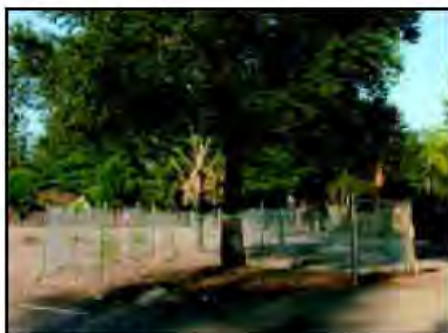
IMAGE 2.15-2 Tree Protection Fence at the Dripline
