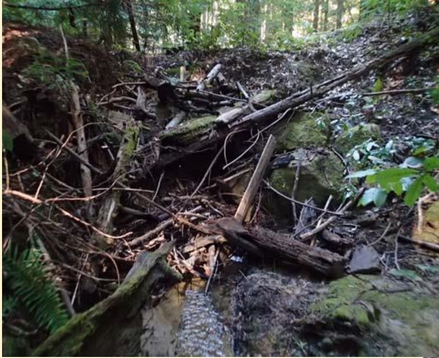
Plugged Culvert
