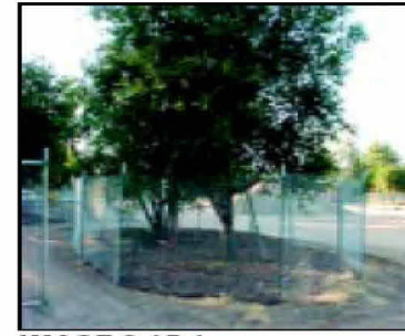
IMAGE 2.15-1 Tree Protection Fence at the Dripline
