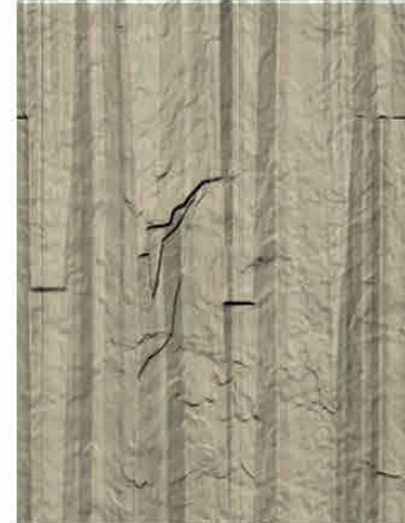
CONCRETE WALL FINISH: BASALT LINER STAINED
