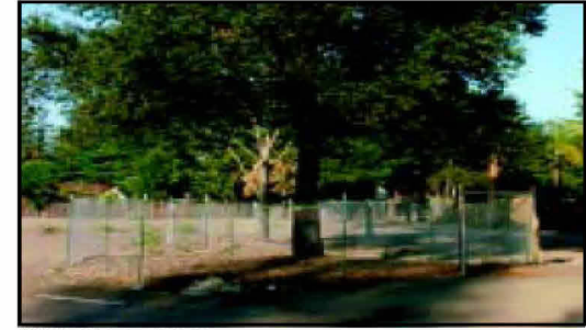
IMAGE 2.15-2 Tree Protection Fence at the Dripline
