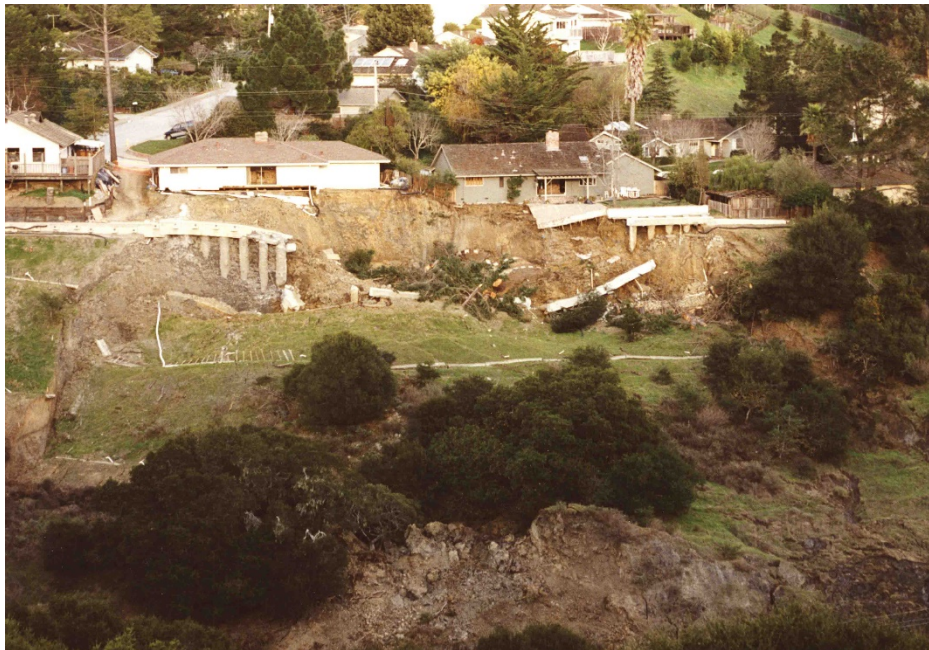
Figure 11 Polhemus landslide behind 1406 Rainbow Drive which blocked Polhemus Road.
