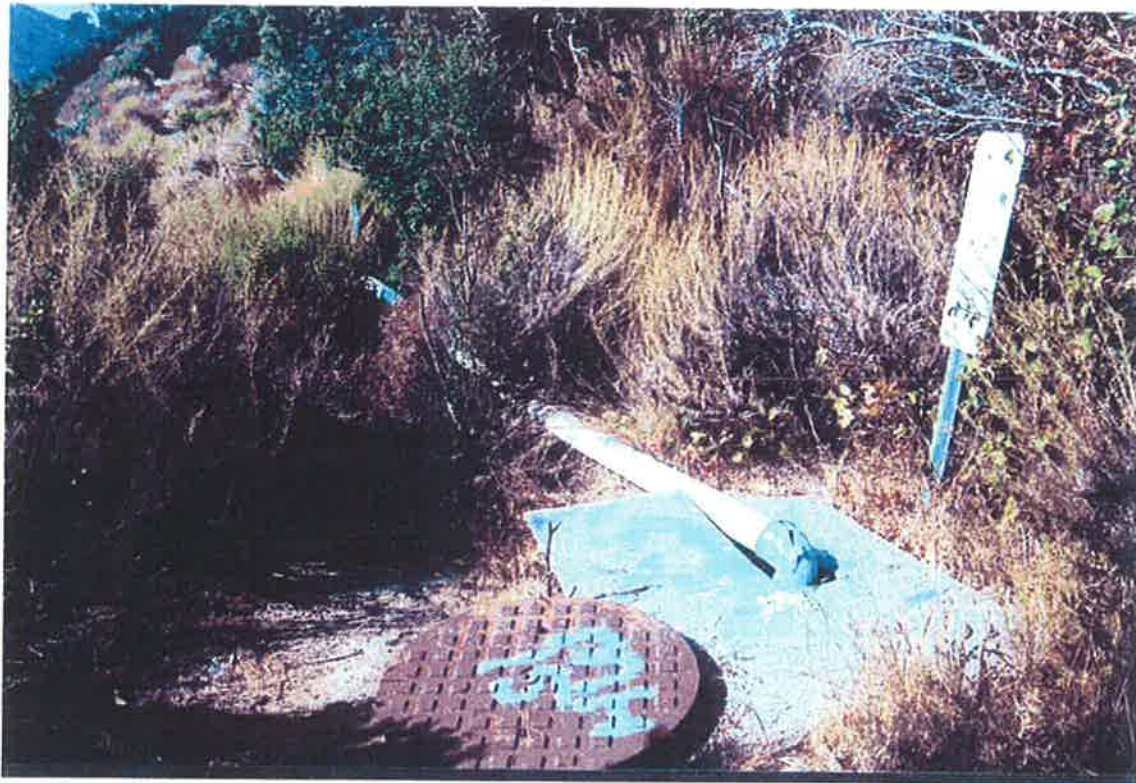
Temporary Bypass Pipe from MH 17 entering MH 15
