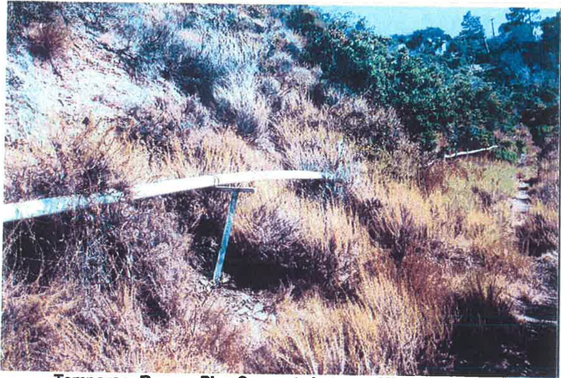
Temporary Bypass Pipe Supports between MH 15 and MH 17
