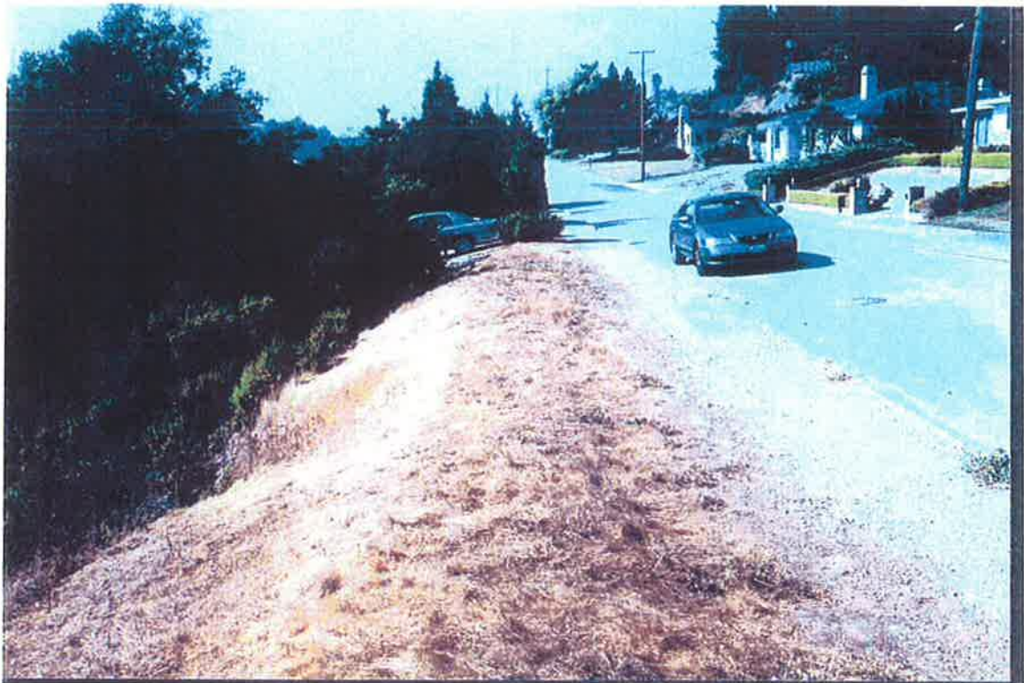
Main Lift Station Site approximately 30 feet left of MH 20 (in street)
