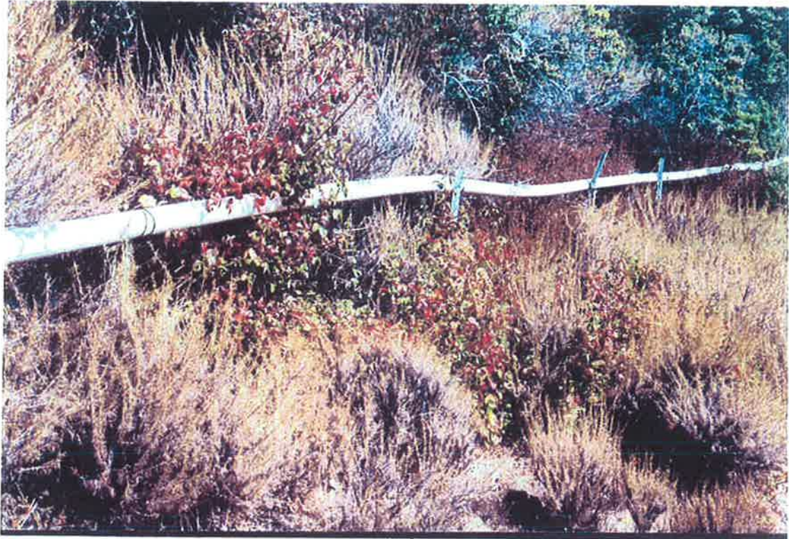
Temporary 4" PVC bypass pipe installed below Parrott Drive
